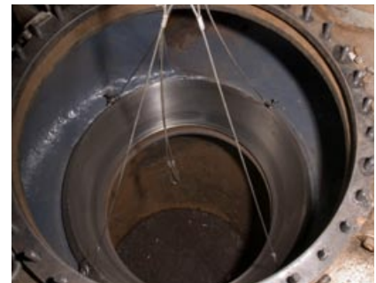
New impeller liner is installed
